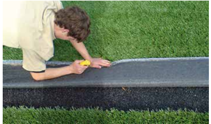
➤ Joint edges to be cut
