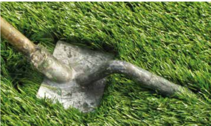
➤ Straighten the turf for optimal optic and performance
