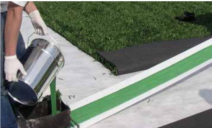
➤ Pull the seam tape through adhesive machine
