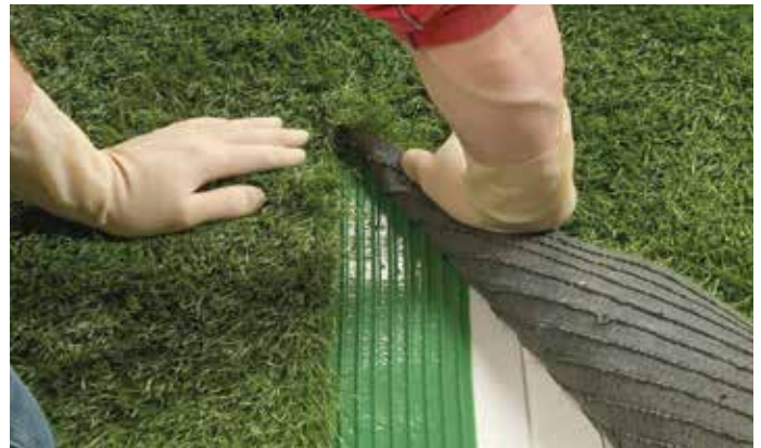
➤ Align the turf with the seam tape
